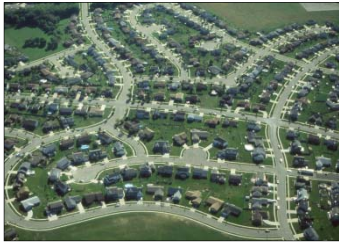
A dysfunctional, discontinuous and confusing road system.
