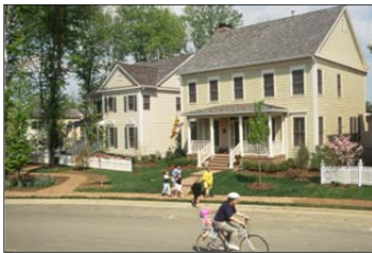
An example of a Build-to line. Notice how front wall of houses remains in-line while the street
