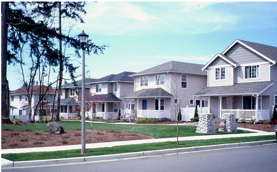
Figure 21: Illustrative example of houses fronting on a park (Not currently provided for)
