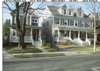
An example of a Build-up line. Notice how eave line is same on both buildings and how change in roof orientation to the street reduces the mass and scale of the building on the right.
